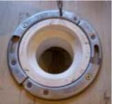
Step 1: Remove corroded steel ring.
